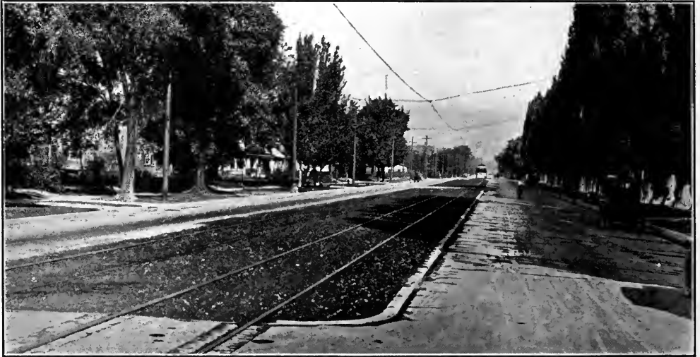
VIEW ALONG 7TH EAST STREET, SHOWING NEW PARK AREA FORMED BY MOVING STREET RAILWAY TRACKS
